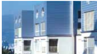
MONTAFORM® Residential development, Olten (CH)
