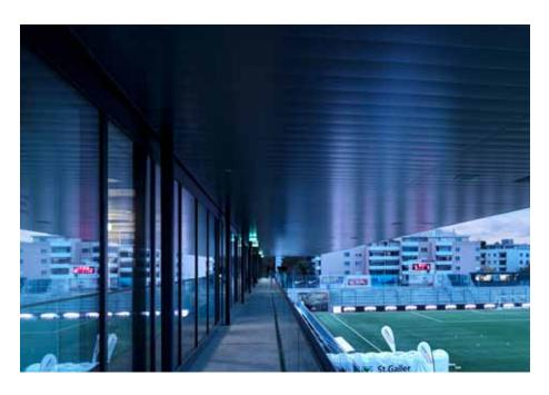
The delicate design of the steel sheets with their closed joints allowed the fast and economic top to bottom assembly using the MONTA-FIX® fastening system and rustproof flat-head screws. Due to the high degree of pre-fabrication of the metal profiles, the number of deliveries to the building site was also reduced.
