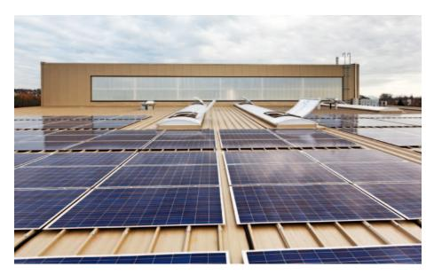
The fire-protection requirements and those in keeping with energy needs also had to be taken into account. The sandwich elements have a U-value of under 0.23 W/m²K and thus comply with that specified by the SIA. This means proof is on hand not only of the thermal insulating property of the composite panels but that they also provide effective heat protection on hot days in summer.
