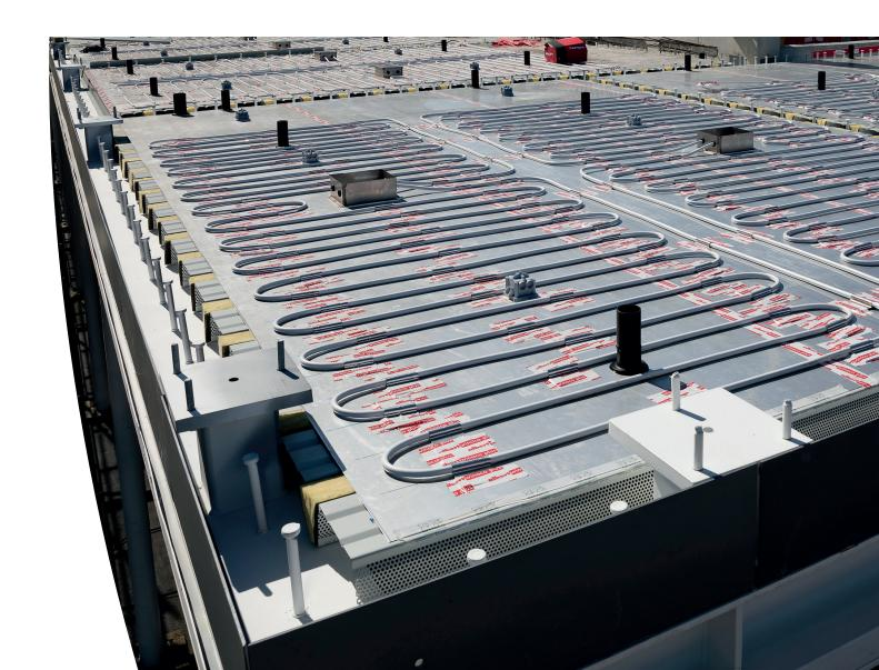
The on-site prefabrication took place over a period of several weeks. After that, the bulky modules were transported with a special jig to a location close to the crane and from there lifted into the steel structure of the Cubic. Following the fastening, sealing and connection of the individual floor fields to form a complete floor system, the last step for the integration of the individually developed and manufactured intermediate floors took place with the concreting over of the modules.
