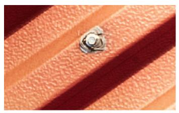
Damaged fastener on roof cladding.
