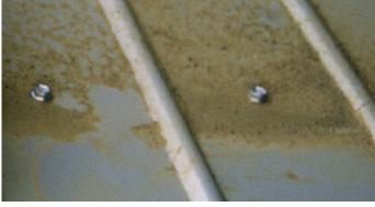
Mould growth on pre-finished steel cladding.
